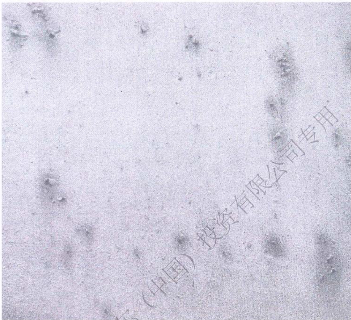
Figure 3 — Degree of rusting Ri 3 *****To be continued*****
